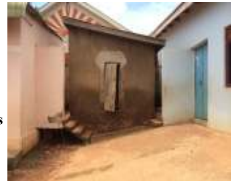
The center (dark) building is the current toilet facility at the school. Boys to the left. Girls to the right
